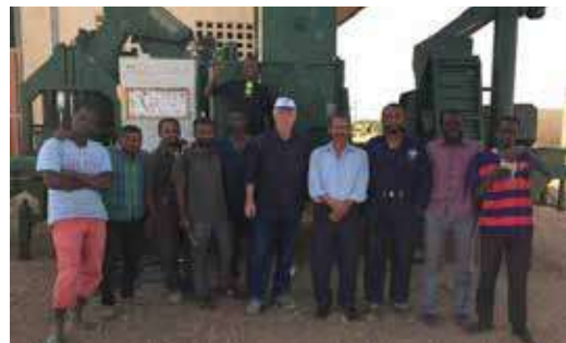
Finishing installation of the machine.
